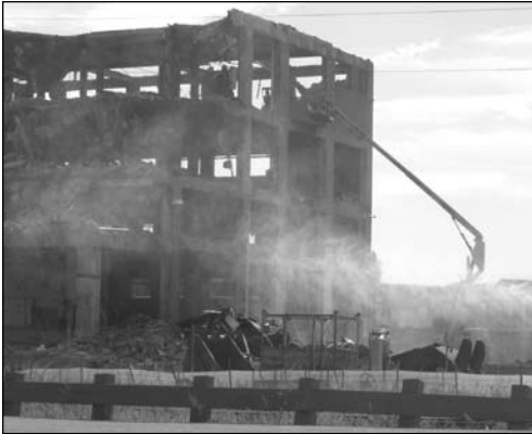
Purina Mill demolition, 2010
